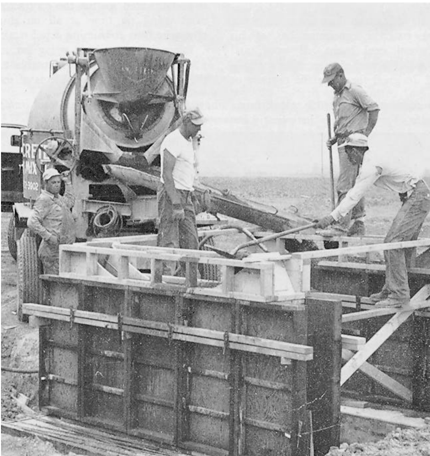
Illustrated is another type of modern prefab form, which features wooden frame and steel cross members.
