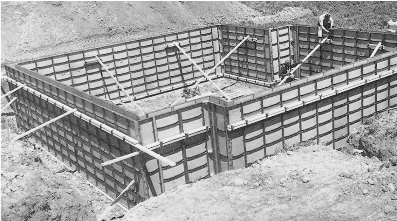
In contrast to the crude plank forms above, this illustration shows steel-frame prefab forms in place for pouring basement.
