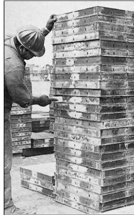
Maintenance of forms can be a tiresome task, but well-maintained forms mean more reuses.
