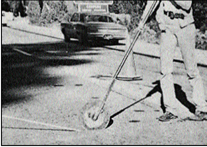
The bond breaker is inserted into the clean joint just before sealing.
