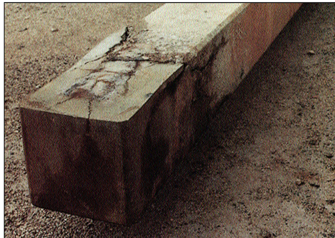
Figure 5. The nonconductive material used to repair this beam (top) accelerated the corrosion of reinforcing steel, which led to premature repair failure (bottom).
