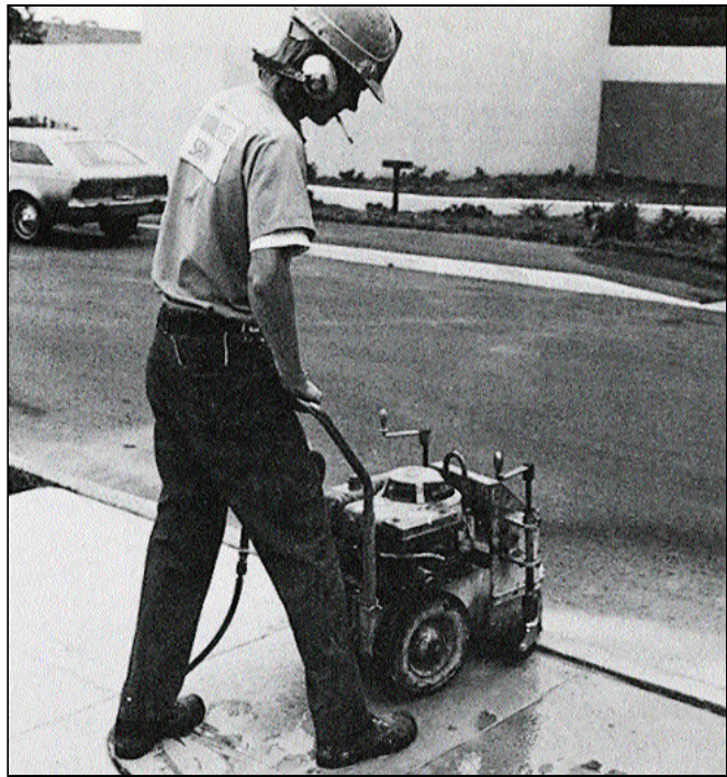
Figure 3. This concrete curb was higher than the adjacent slab and could have caused trip-and-fall accidents. A machine with a diamond grinding wheel was used to grind down the protruding curb.
