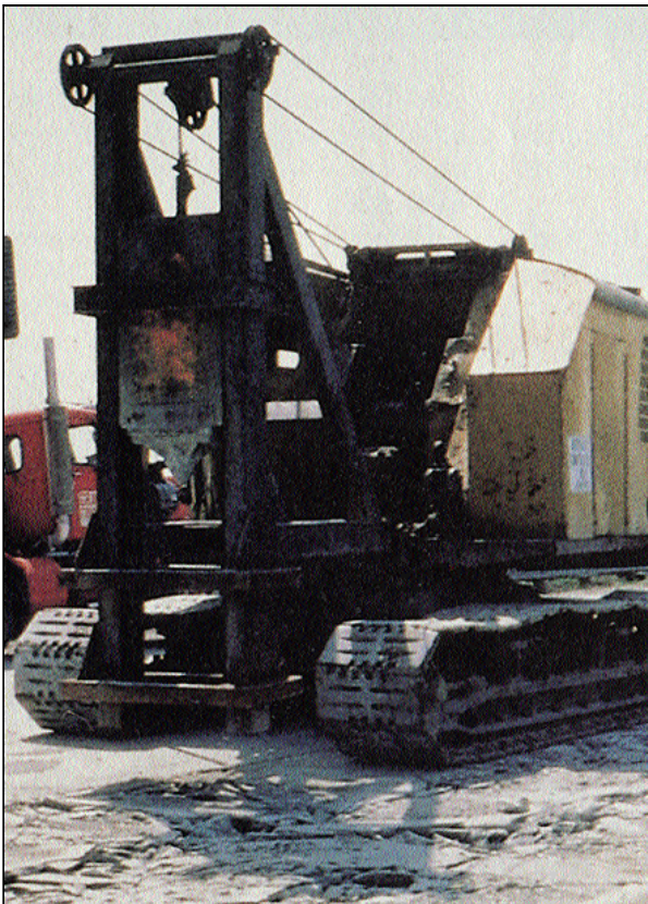
Figure 1. Early pavement recycling jobs used a drop-weight type pavement breaker.
