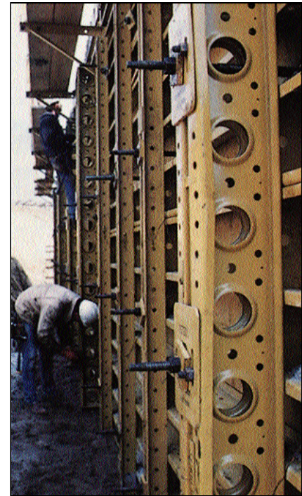
Figure 3. Pre-formed holes in the channel webs and flanges of these steel beams allow easy insertion of bolts, form ties, and other connections.
