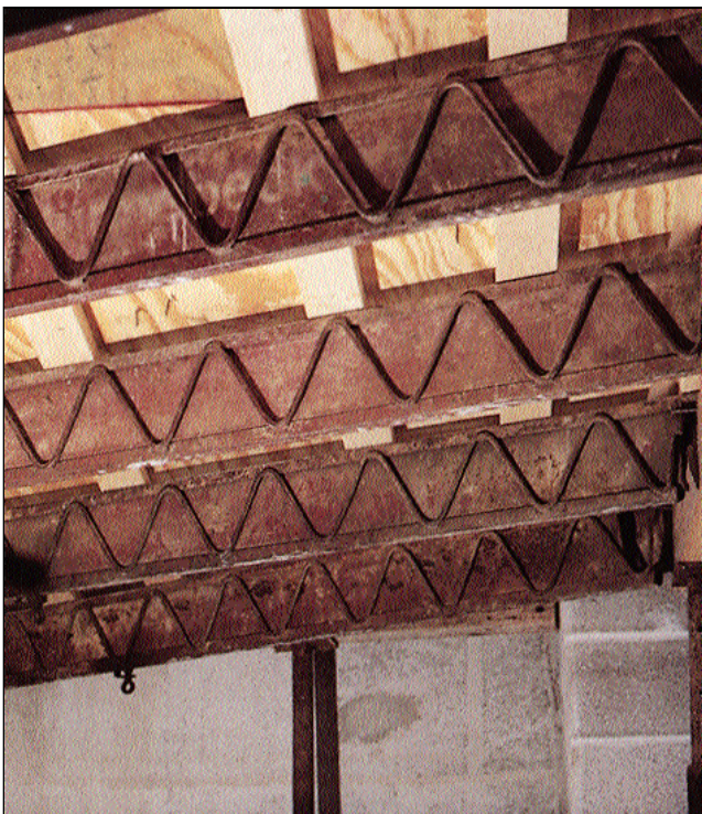
Figure 4. Used as joists under plywood sheathing, adjustable horizontal shores can support deck spans as long as 20 feet without intermediate vertical shoring. An I-beam or plate section telescopes to the desired shore length from an outer lattice member or box-beam.
