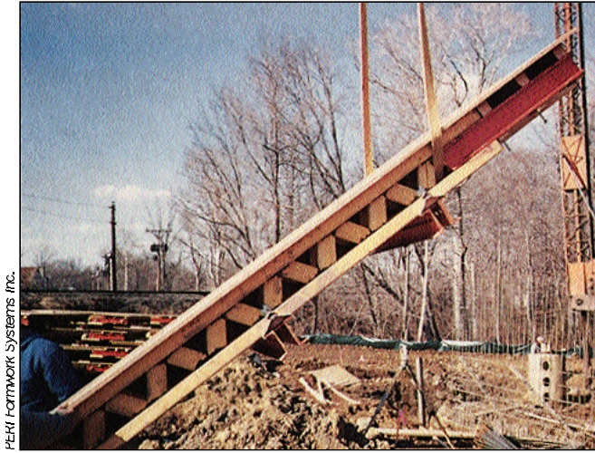
Figure 2. Wood girder has a lattice truss section that adds strength and simplifies waler alignment. Here a preassembled wall form panel using the girders and steel walers is being hoisted into position.
