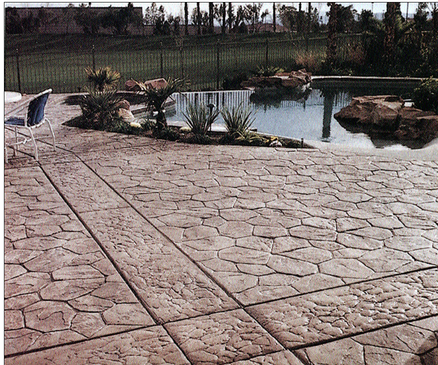
This concrete pool deck was created using two different random-stone patterns. The bands of small random stone break up the expanse of larger stone to create visual interest and define areas.
