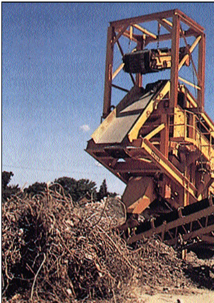
Figure 2. Final removal of steel (typically dowels and tie bars) takes place at the recycling plant during crushing. An electromagnet catches steel moving along a conveyor belt between primary and secondary crushers. In the foreground is a pile of steel removed during crushing operations.
