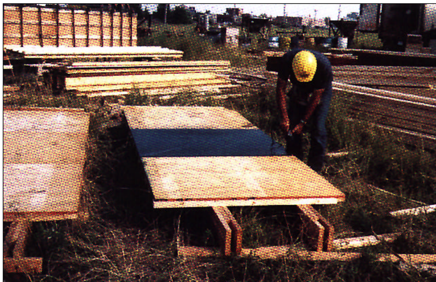
Figure 4. Plastic lining is commonly attached to plywood forms to provide the durability necessary for slipforming structures taller than 200 feet.
