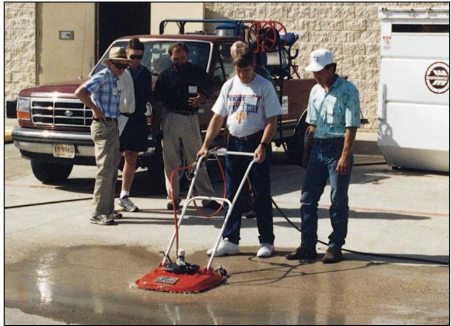
Figure 2. Wheel-mounted power-washing units increase cleaning speed on large horizontal surfaces.
