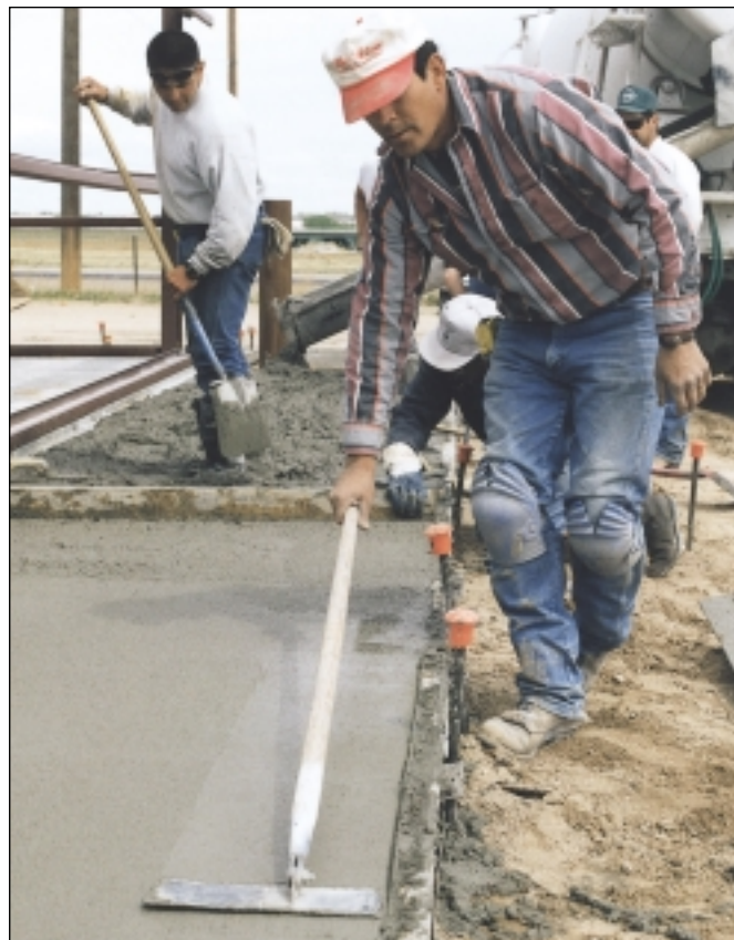
Above: Darbies serve the same purpose as bull floats except they are used on smaller areas and are moved across the concrete surface in a sawing arc instead of a back-and-forth motion. Right: If you prefer to stand while edging, use a walking edger that attaches to a long handle. One type of handle bracket allows you to flip-flop the handle to either side of the edger. Another type (shown here) locks the handle in a set position.
