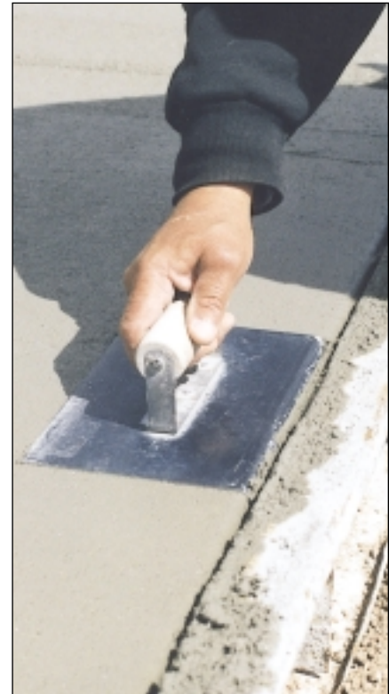
Above: When using a bull float, keep the leading edge of the blade slightly inclined above the slab surface. Right: To create a neat, rounded edge, run the edger back and forth with the leading edge slightly raised.
