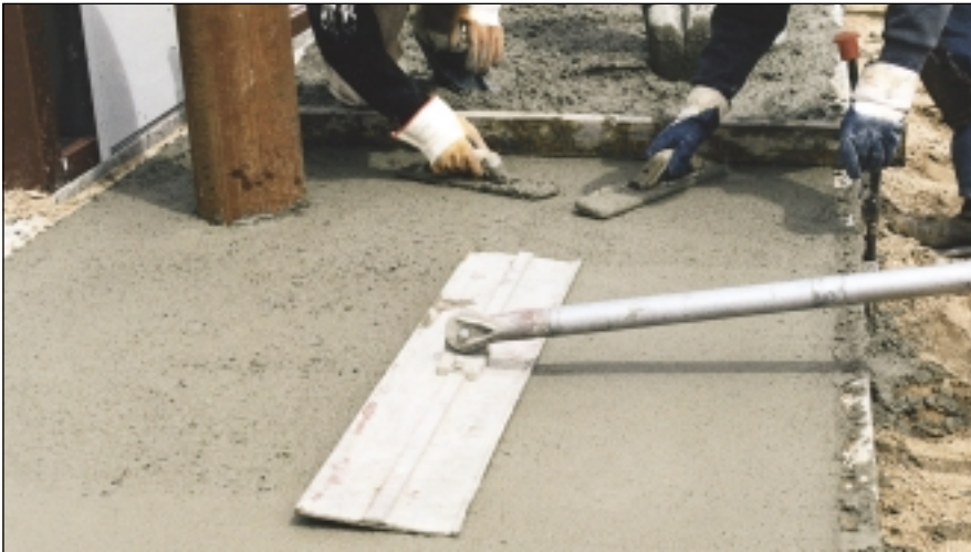
Above: When using a bull float, keep the leading edge of the blade slightly inclined above the slab surface. Right: To create a neat, rounded edge, run the edger back and forth with the leading edge slightly raised.
