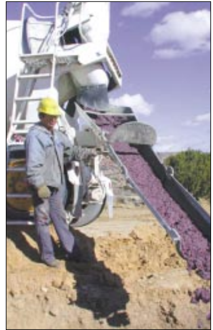
Purple flowable fill is placed in a utility trench in New Mexico.
