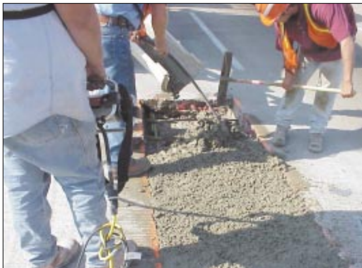
Above: A typical restrained deck repair patch has cracked and is marked for replacement. Left: The construction crew places a repair patch on a bridge deck.
