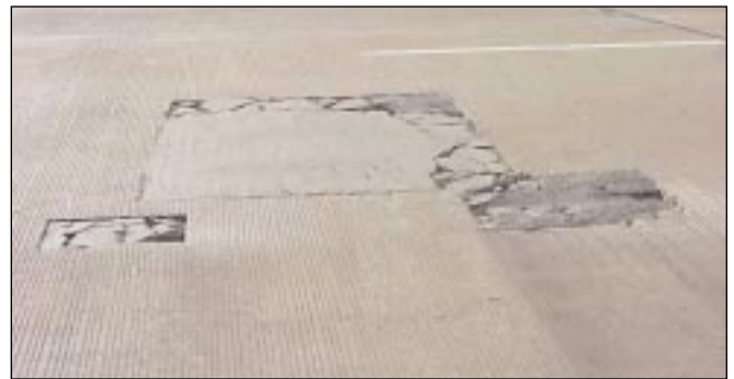
Above: A typical restrained deck repair patch has cracked and is marked for replacement. Left: The construction crew places a repair patch on a bridge deck.
