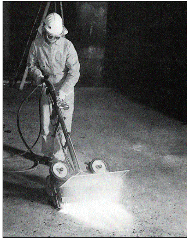
This flame-treating unit moves forward by means of a chain drive operated by a hand crank. Pressure gages and flame controls are on handle.
