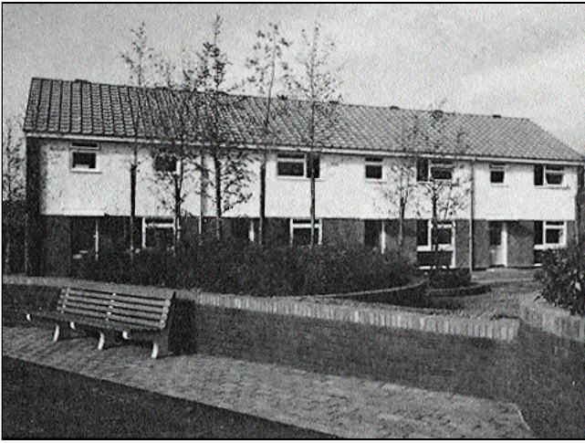
Two-story no-fines homes in Eastfield Estate, Scarborough.
