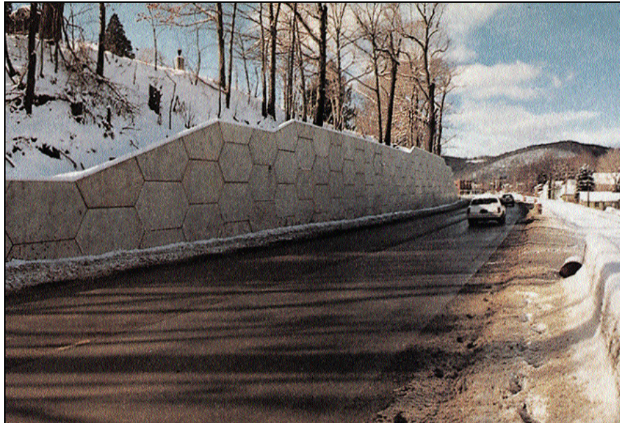
Constructed from the top down, a ground-anchored wall is especially suited for cuts. The wall face can be shotcreted, cast in place, or (as shown here) precast.
