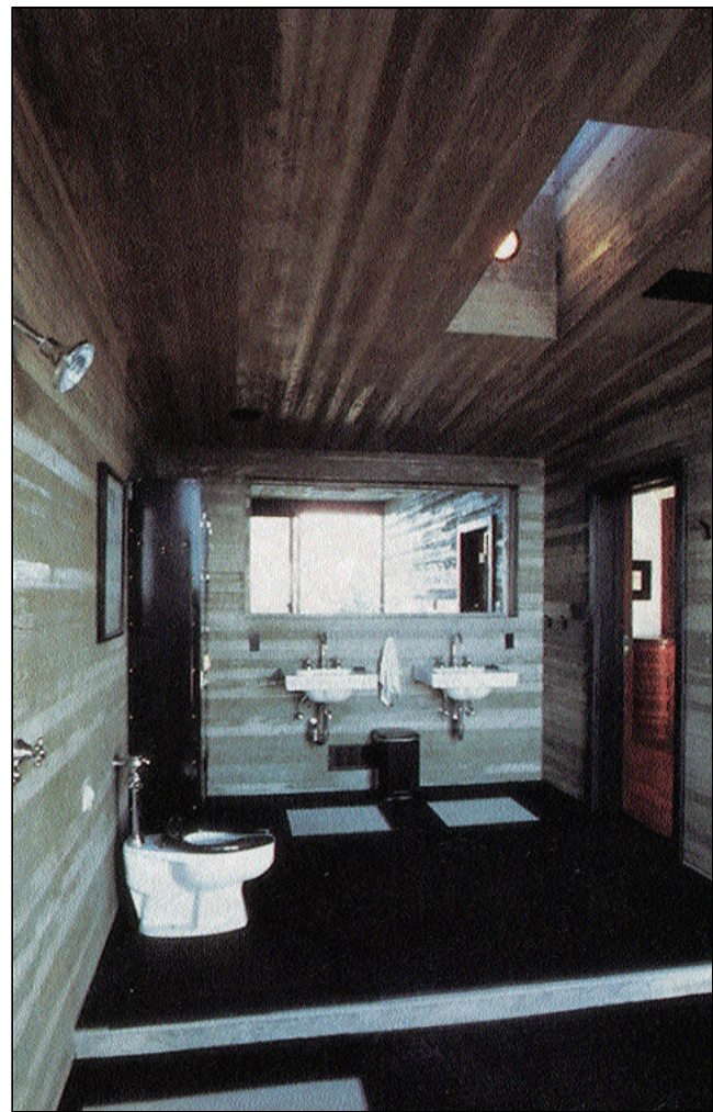
Black vinyl duckboard flooring and a floor drain allow this concrete bathroom to be hosed down for easy cleaning.
