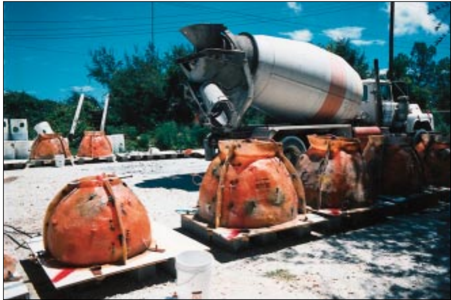
Fiberglass molds set up for production in Charleston, S.C.
